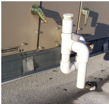
CONDENSATE P-TRAP (always required)
